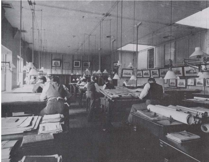
**Figure 1.3:** An example of the amount of space available in traditional work spaces. Large drafting tables are surrounded by documents and blueprints. Much space is available for viewing and recording information. The photograph, from Ferguson [Fer92], is of the drafting room of Baltimore & Ohio Railroad, 1899.
